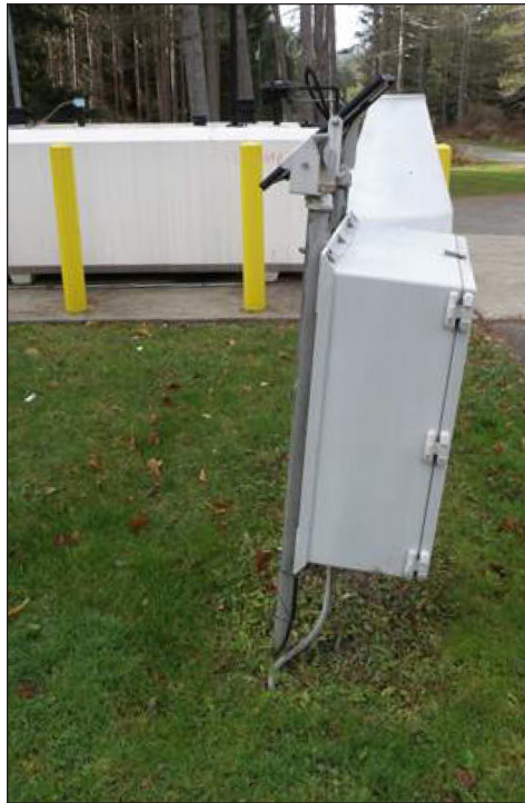
Figure 3: A Damaged Precipitation Gauge Used by the National Weather Service (NWS) That Was Not Repaired as of Fiscal Year 2016
